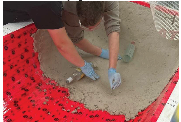
Figure 7. Glass Bottles Smoothing Concrete and Painted Nails Verifying Thickness
