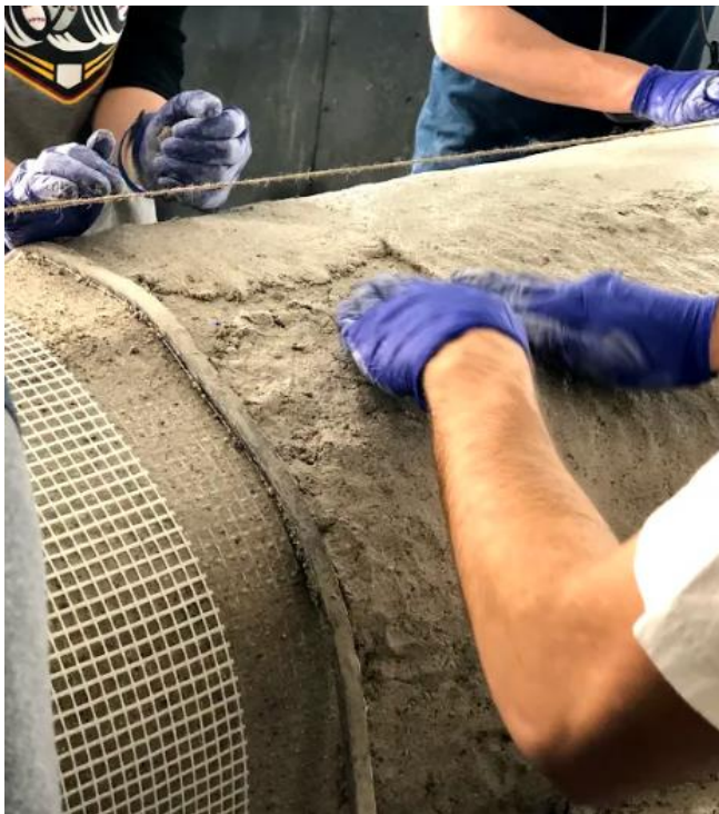
Figure 4. Concrete placement and layering scheme on casting day for KEPLER [8] .
