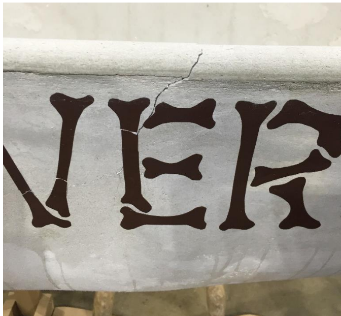
Figure 7: EXTINCTION Structural Crack
