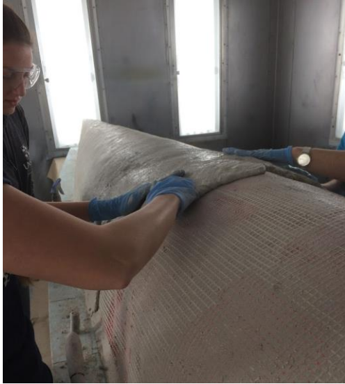
Figure 14: Placement of concrete layers
