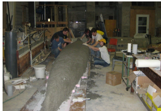
FIGURES 4 & 5: CNC ROUTING OF THE FORMWORK AND PLACEMENT OF MAIZIN' RACE
