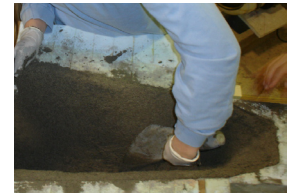
Figure 18: Finish Placement
